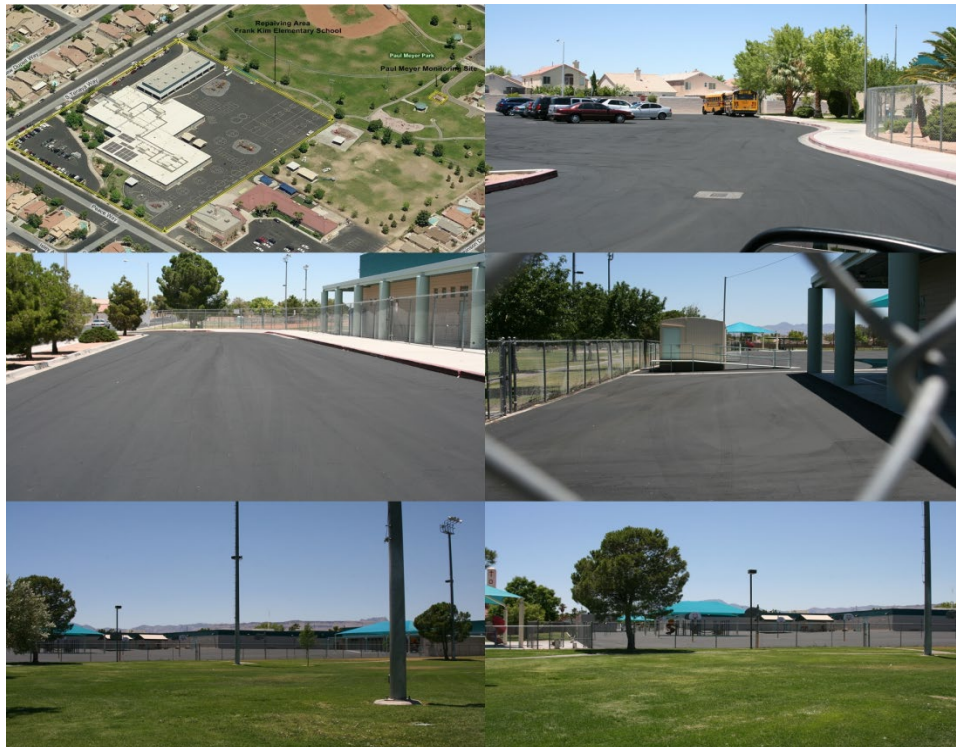
Figure 13. Paving Operations Adjacent to Paul Meyer Site on June 21.
